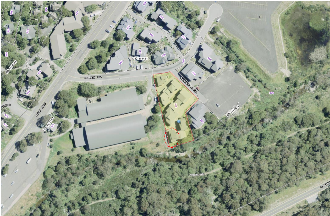
Figure 3: Aerial view of the subject building in context of the locality
